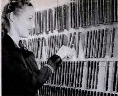
Recorded on 16-mm. motion-picture film, each doctor's code number is encased in a plastic stick. Girl above lifts stick off a filing board to put it on the transmitting machine.
